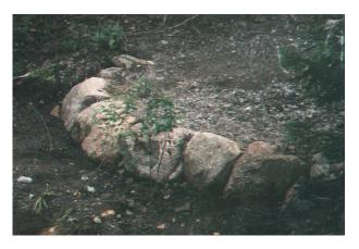
4. A single row of medium sized rocks (less than 1 foot high) might be effective at the waters edge in an area that receives a lot of use and foot traffic, such as where you access the lake or a dock.\* It is important particularly where the groundcover is grass, as grass is shallow-rooted and easily undercut by wave erosion. Install filter fabric behind the rocks so that fine soils do not wash out from behind the rocks.
